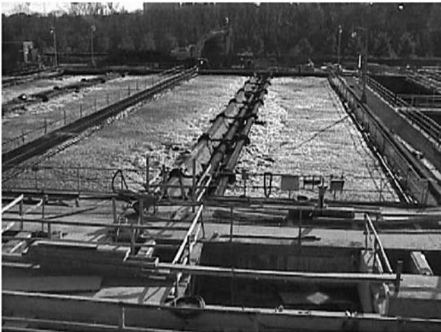
Figure 8.8 Aeration tanks with submerged fine bubble diffuser system (photo by Rumana Riffat).
