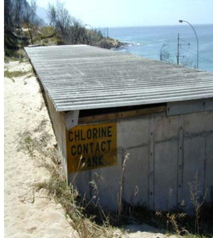
Disinfection of the treated effluent is usually done by dosing chlorine to the treated effluent. The chlorine kills the remaining harmful bacteria and other organisms that are still in the water.
