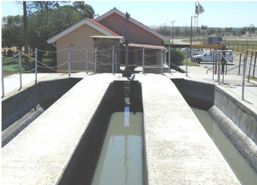
In the primary settling tanks the solids are settled out of the raw sewage, from where the solids (sludge) is transferred to sludge digesters, and the water to the aerobic biological reactors. The main process stream is the aerobic biological process since the liquid component makes out the major portion of the wastewater.
