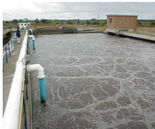
In the secondary settling tanks the humus sludge (or waste activated sludge, depending on the type of reactor) is settled out of the water. Once again the process
