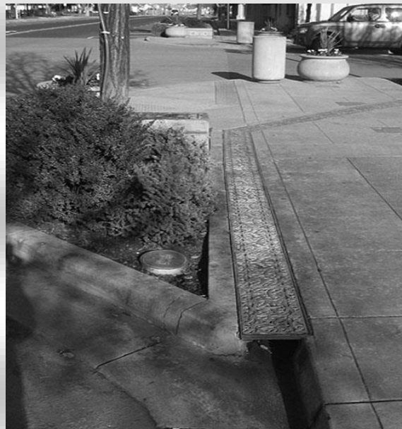
Figure 10.19 Curb extensions may be used as landscaping or hardscape opportunities. This example shows a retrofit curb extension with drainage retained between the extension and the curb. Source: Community, Design + Architecture.
