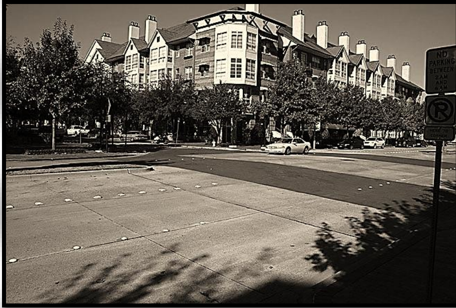
Figure 10.15 Crosswalks with colored bricks contrast with concrete pavement. However, over time, colored bricks stain and lose contrast. Painted stripes marking brick or colored concrete crosswalks would increase their visibility. Otherwise use standard crosswalk markings for long-term visibility. Source: Kimley-Horn and Associates, Inc.
