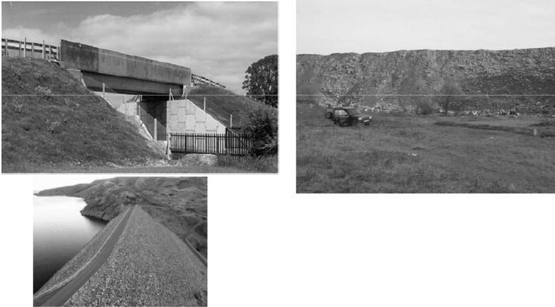
**Fig. 2.1 Embankments and landfills cause to increase subsoil stresses**
